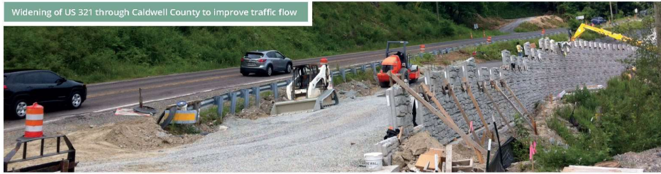
Widening of US 321 through Caldwell County to improve traffic flow
