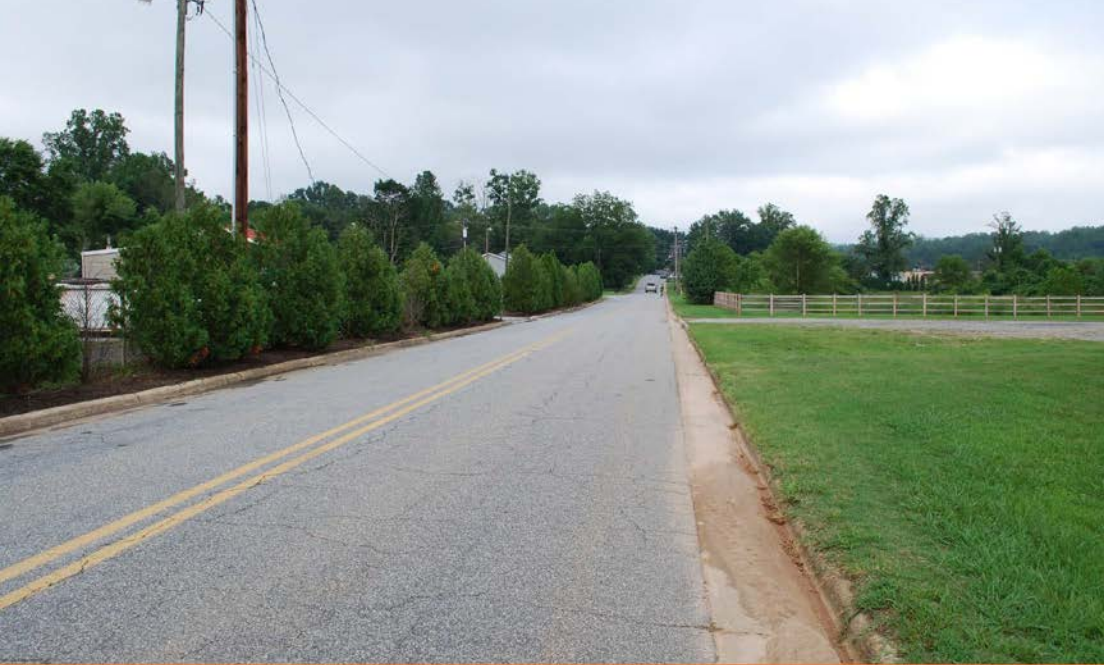
PENNTON AVENUE — EXISTING
