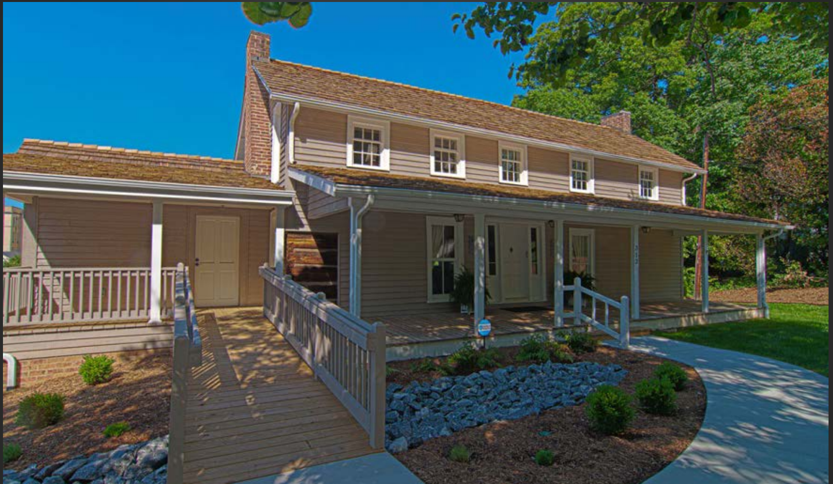
Relocation and Renovation of Rankin House on Ridge Street
