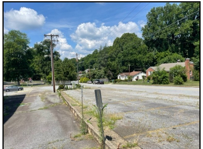
Above: Poplar Street along side of West Lenoir Elementary
