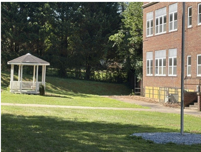
Above: Front of West Lenoir Elementary with gazebo
